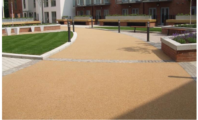
Fig 13- Coloured Asphalt Surface
